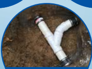
Septic/Sewer Repair & Replacements
